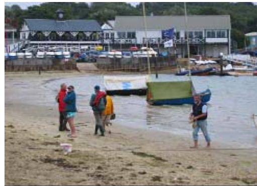
Setting-out for Baywatch restaurant. Picture by Steve Bradwell
